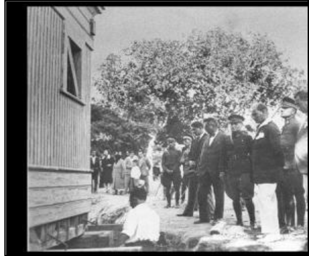
Figure 4. In Yalova, reconstruction of Yeşil Köşk (24 July 1930) [1]
